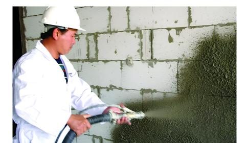
REPCON TI is a single component, polymer modified, fibre reinforced, rapid curing cement based repair mortar to fill the hole REPCON TI is supplied in powder form, ready to use with the addition of water to provide a durable, rapid setting, high strength and easy to apply mortar with excellent low sag properties. Uses:
