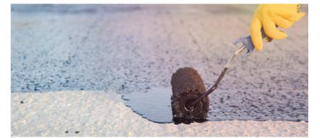
WATERBAR SW is a rectangular acrylic sealing agent. It swells in contact with water to seal all type of construction joints and penetrate in concrete structures.
