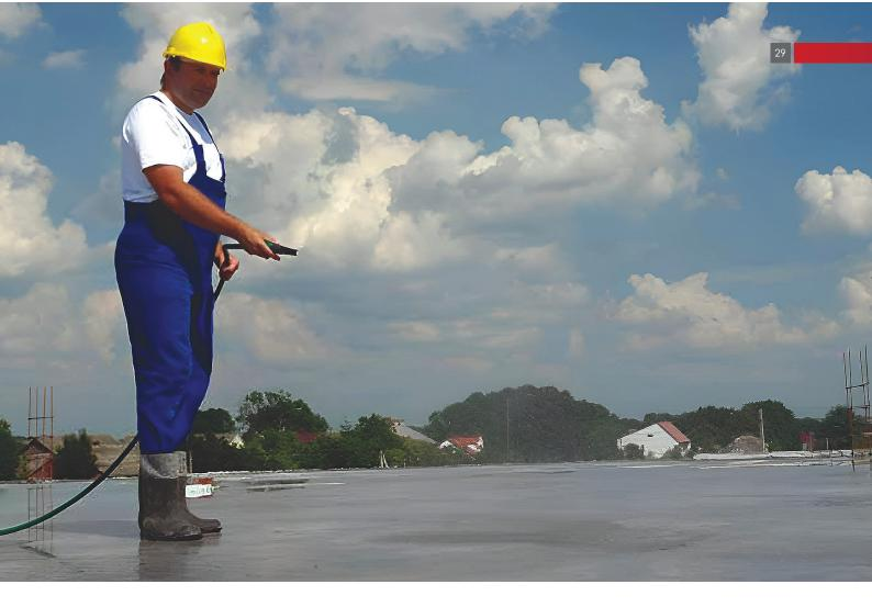
It is not recommended for application when subsequent renders, toppings or coatings are to be applied within the degradation time unless it is removed by cleaning if insufficient time has elapsed to achieve full degradation.
