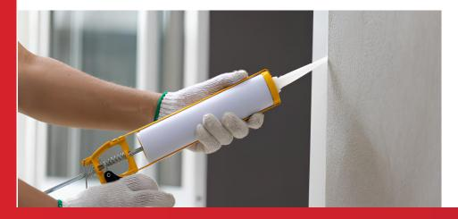
• Gun grade sealants - These sealants are suitable for use in vertical and horizontal joints
